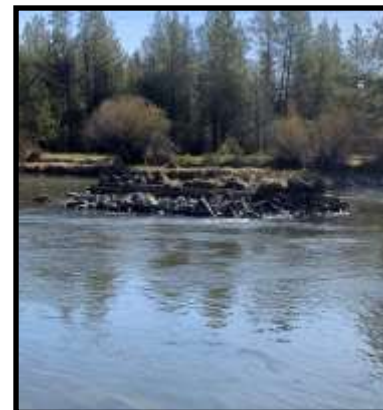
Besson Bridge Remnants, summer 2024 from the West Bank of the River
