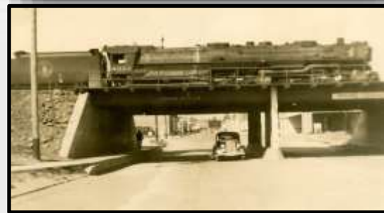
Greenwood Underpass, circa 1940s
