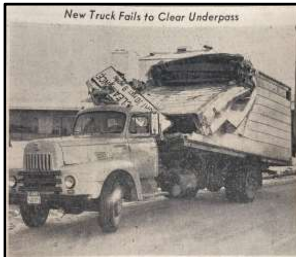
Bend Bulletin, February 20, 1953 Note the bridge clearance sign wedged behind the cab
